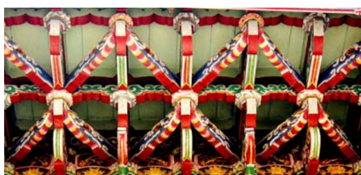
Figure 18. Meshed bracket set in both sides of the Tri-River Hall
