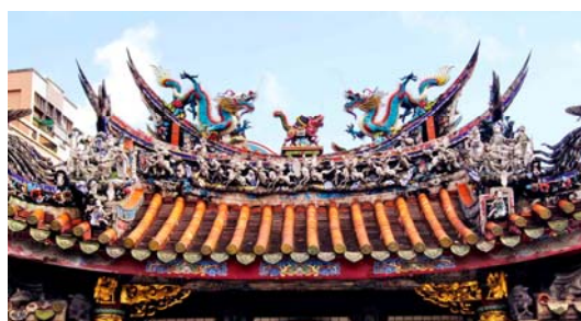
Figure 5. Xieshan style roof of the Dragon and Tiger Gates
