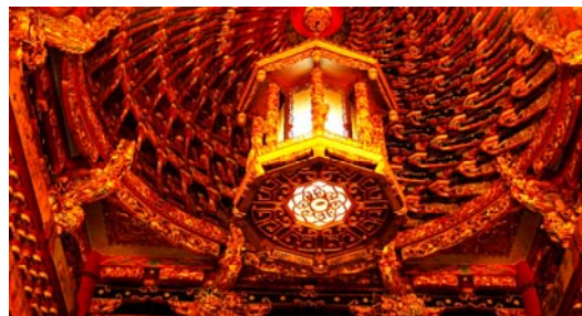
Figure 11. Spiral caisson ceiling of the Main Hall
