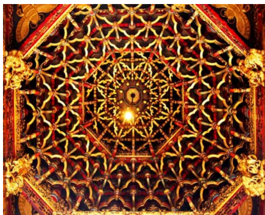
Figure 19. Octagonal caisson ceiling
