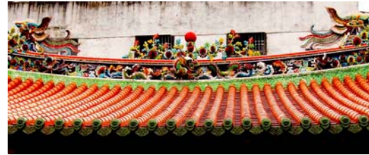
Figure 12. Yingshan style roof with single-tiered eave of the Rear Hall
